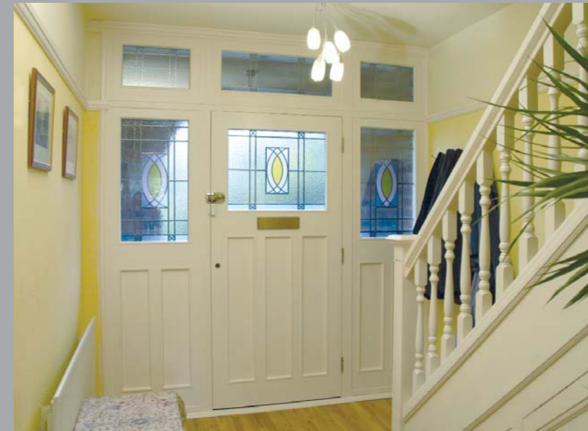
BESPOKE DOORSET WITH SIDELIGHTS AND STOREY FRAME
